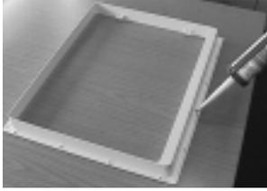
1. Seal the mounting frame, making it waterproof.
